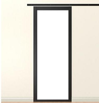
6. Use a pencil to mark the wall 1.7 inches above the door. This mark is where the rail will be installed.
