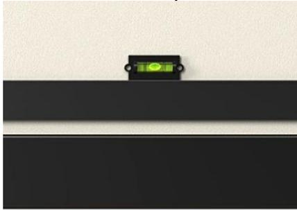
8. Line up the rail with your marks from steps 6 and 7. Use the included spirit level to make sure the rail is straight. Mark the positions of the holes with a pencil.
